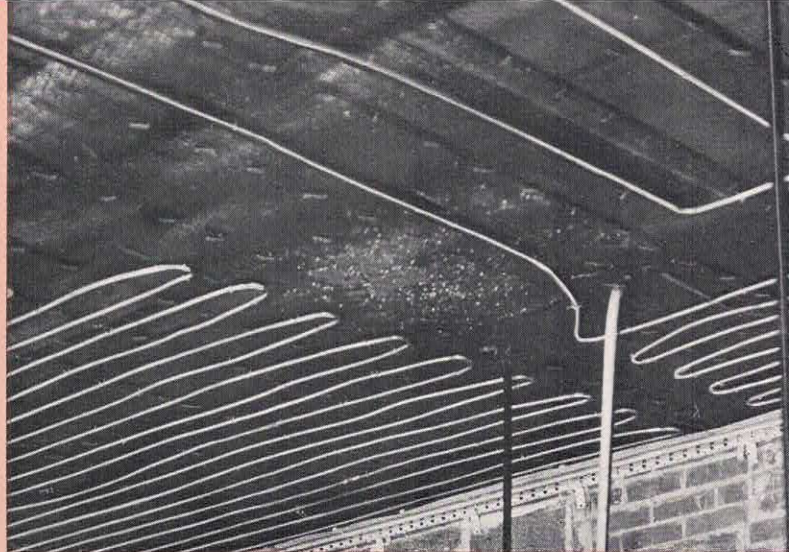
For most installations, the copper tube used need not be large in diameter; hence the plaster covering in a ceiling or wall panel will not be excessive.
